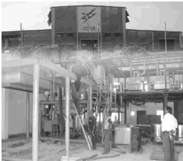
The biomass based gasifier unit managed by the CBOs
